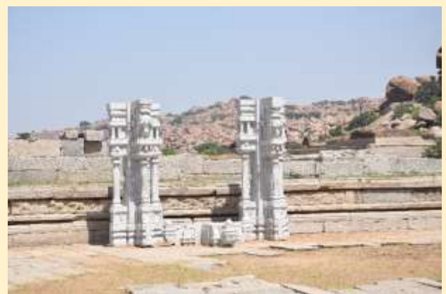
New pillars to restore- rejected by Unesco?
